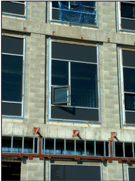
UBC Life Sciences Building – Brick Veneer over Block Backup
