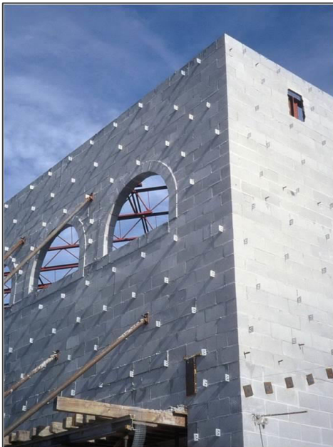
Typical rain screen wall assembly – block backup
