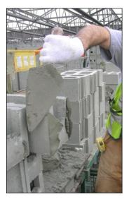
Mortar joints being "Tooled" after several courses have been are laid
