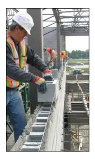
Mortar being spread on the vertical "Head Joint"
