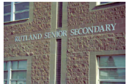
Combination of coloured splitface with natural smooth units framing the windows and half-high smooth in vertical recess.
