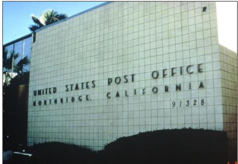
Reinforced Block Structure
