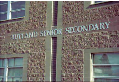
Combination of coloured splitface with natural smooth units framing the windows and half-high smooth in vertical recess.
