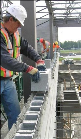
Mortar being spread on the vertical “Head Joint”
